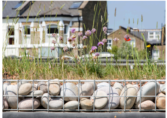
Figure 2.4 Retrofitted biodiverse green roof
