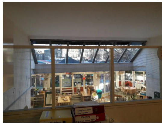
Window ceilings on top floor
