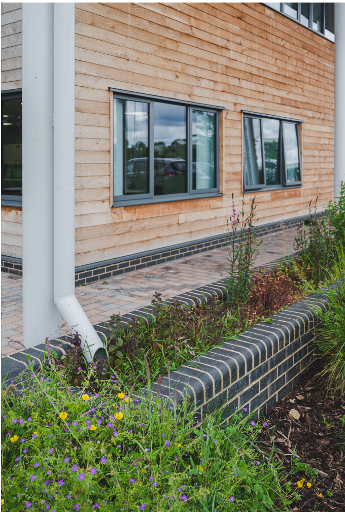
Figure 3.1 Raised wetland receiving rainwater
