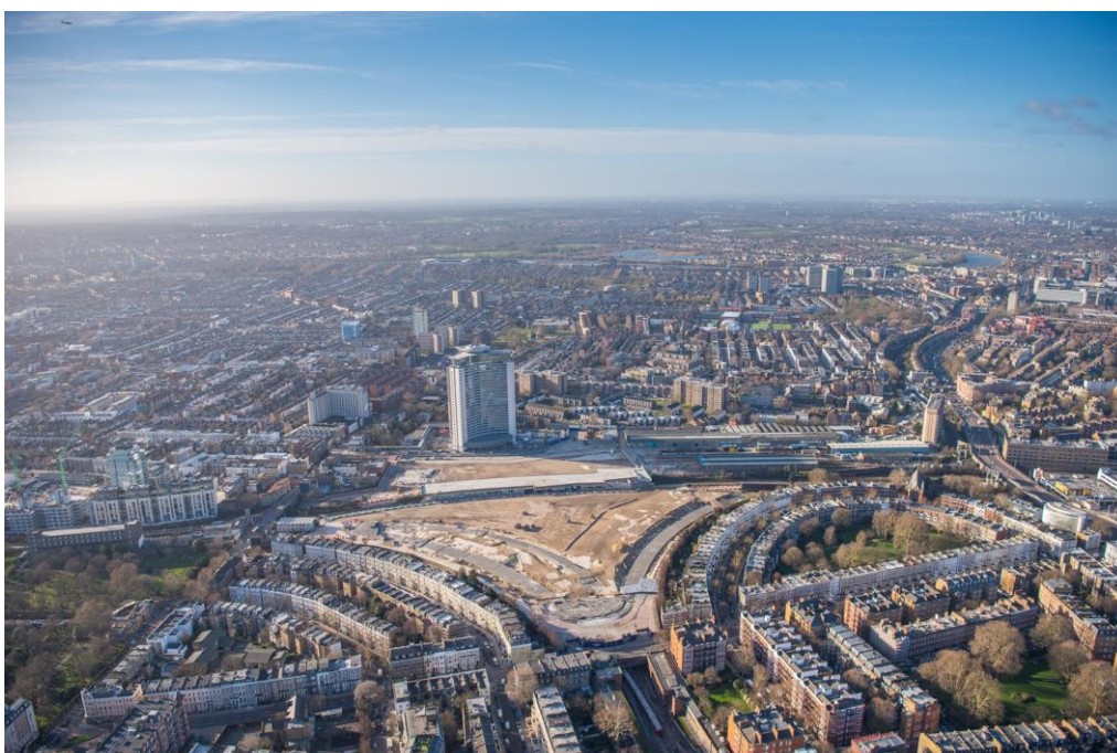
Fig. 3: View of Earls Court masterplan site looking west
