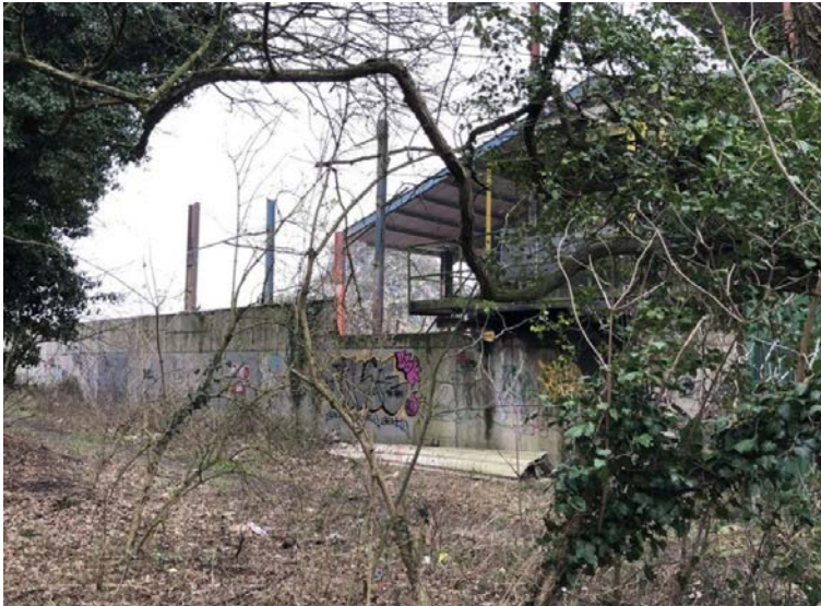
4. Buildings facing the canal at the waste transfer station
