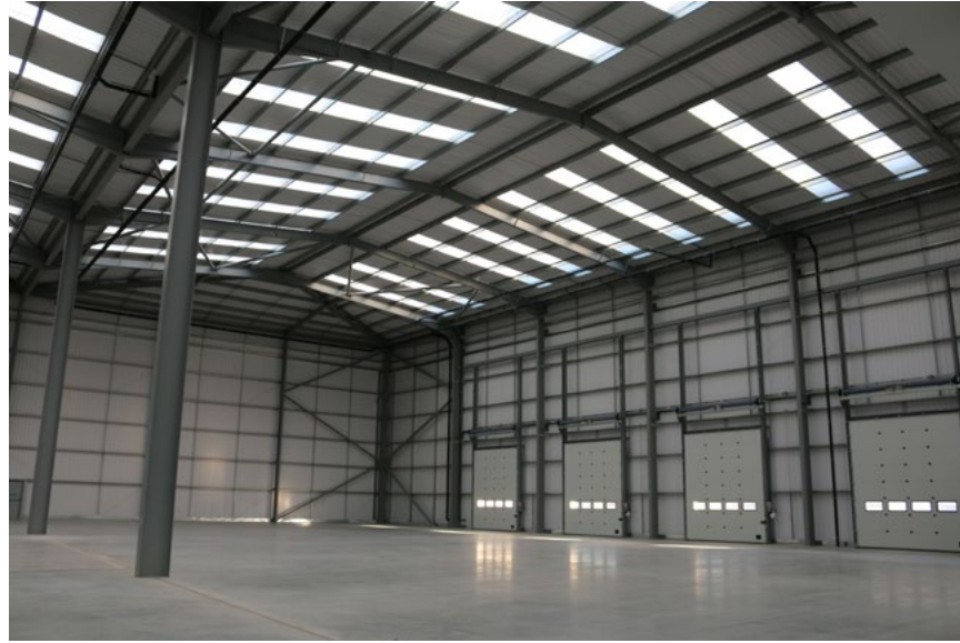
Single storey - Steel frame Unit 2, Origin, Park Royal, Segro
