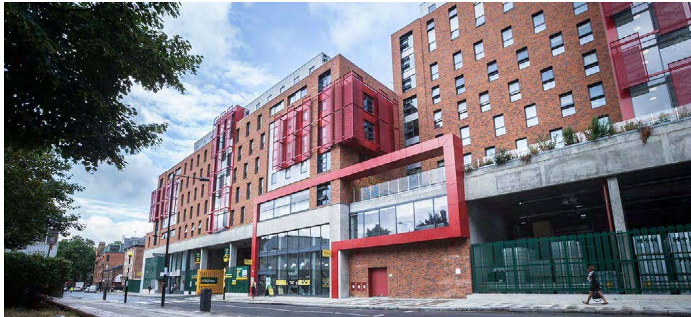
Mixed industry - residential - Concrete frame Travis Perkins Kings Cross, Cooley Architects
