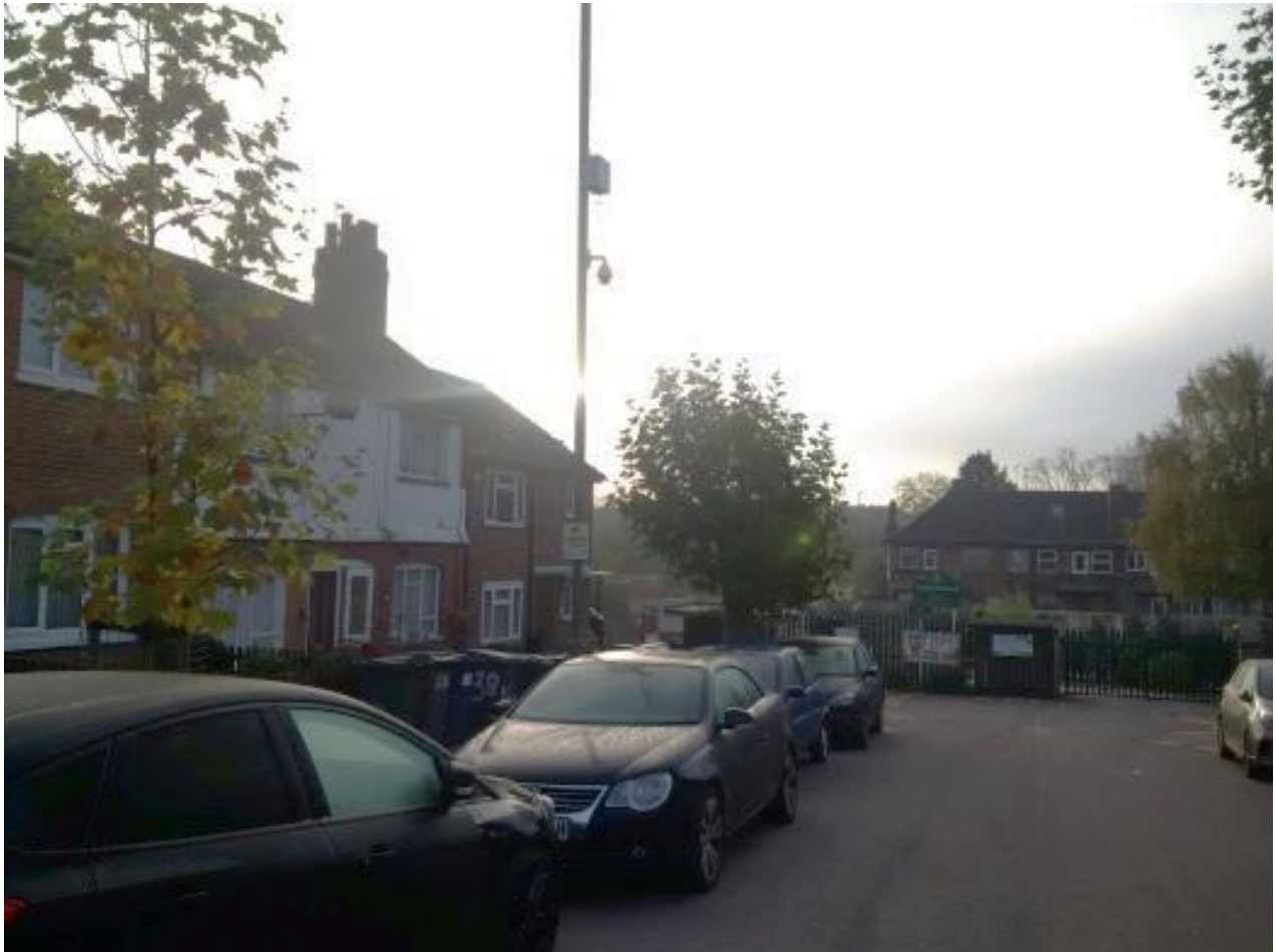
CCTV and zig-zags at Queen Road
