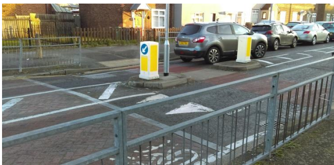
Raised table (but no formal crossing) for pedestrians to cross Goresbrook Road, connecting the school with The Gores
