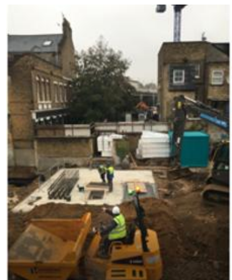
Construction site opposite
