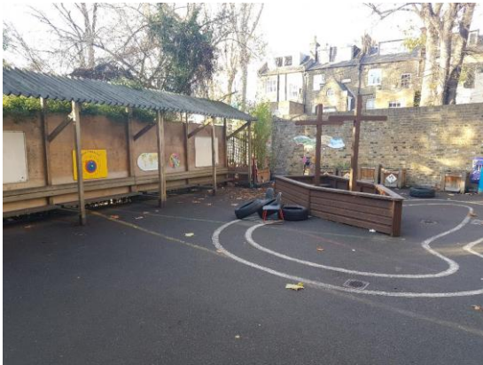
Playground adjacent to school building
