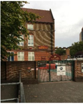
School entrance space set back from Oxestalls Road
