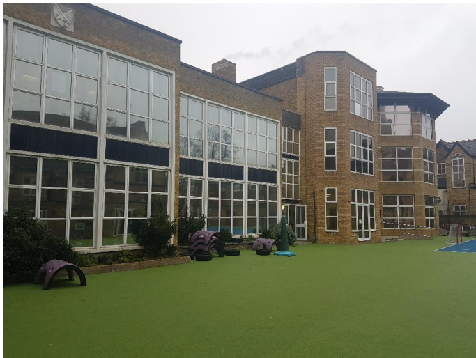
Broadway Site – Older building
