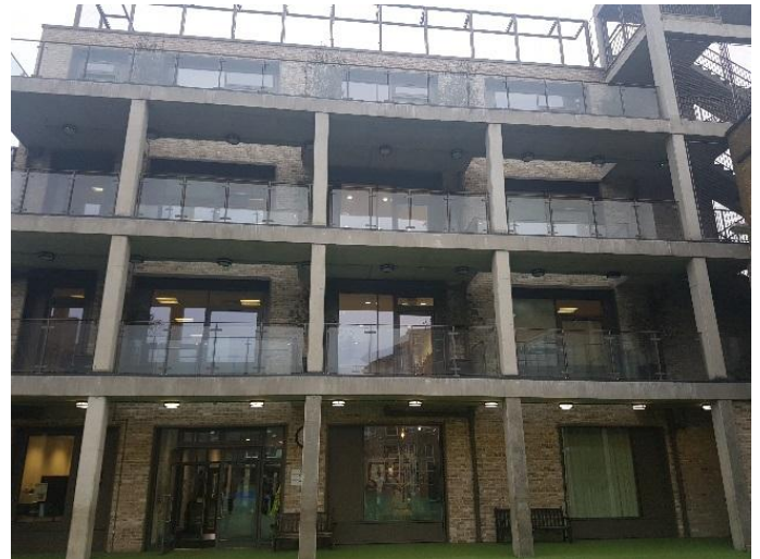
Broadway Site – New building
