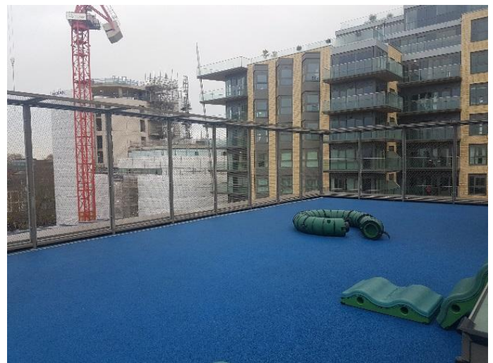
Broadway Site – Rooftop playground
