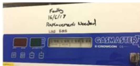
Broken heating equipment. Note reads 'Faulty 16/6/17 Replacement Needed.'
