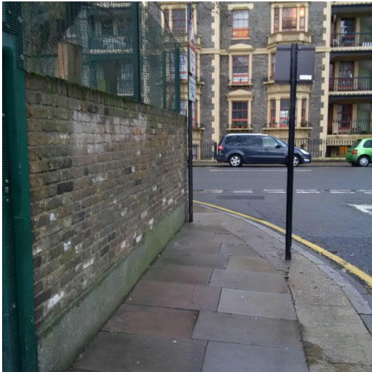
Wide bell mouth Pelter Street and inadequate drop crossing provision
