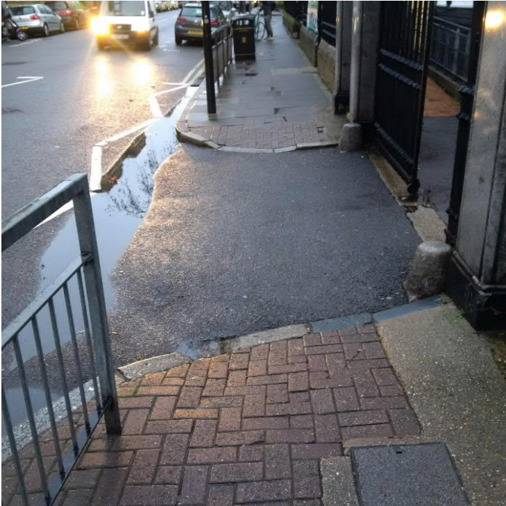
Former and unused vehicular crossover and guard railing
