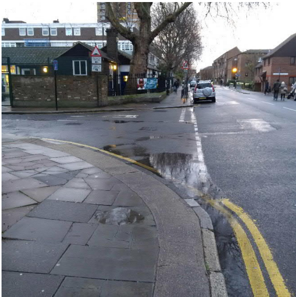
Wide bell mouth Pelter Street and inadequate drop crossing provision
