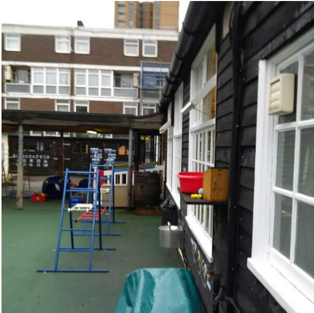
Boiler flues, wooden construction of building and opening of windows in December
