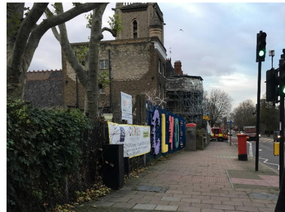
A200 Evelyn St (NW Bound) – Nursery perimeter fence and adjacent pedestrian crossing
