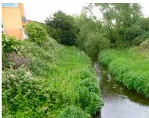
Flood relief channel (8)
