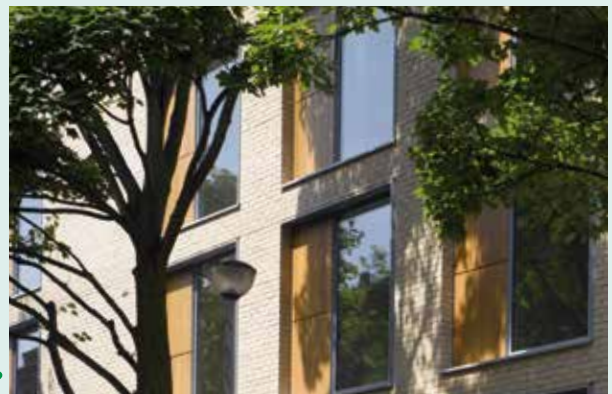
Window brick reveal is to be a depth of 1 brick (215mm)
