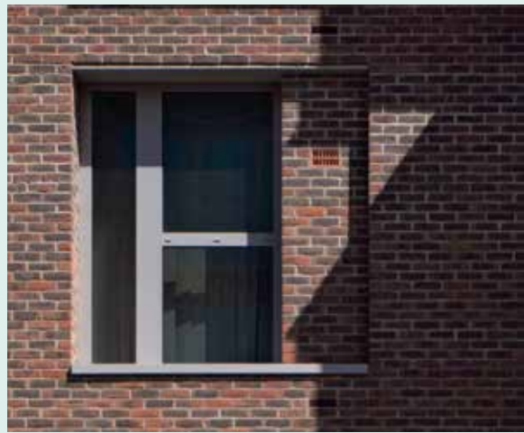
IF residential window brick reveals to be a depth of 1.5 bricks (327.5mm)
