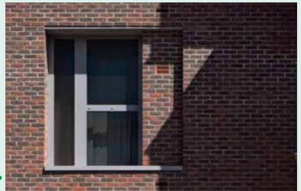
Window brick reveals to be a depth of 1.5 bricks (327.5mm)
