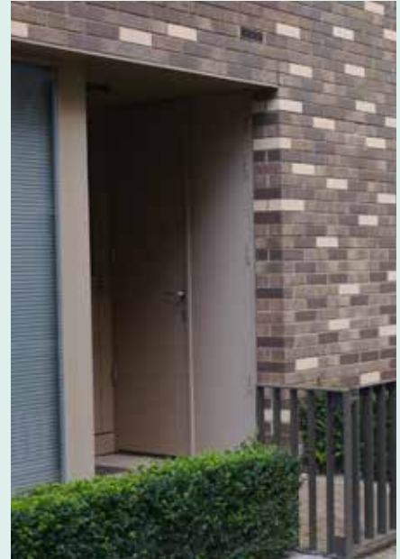
Concealed metres and controls ✅
