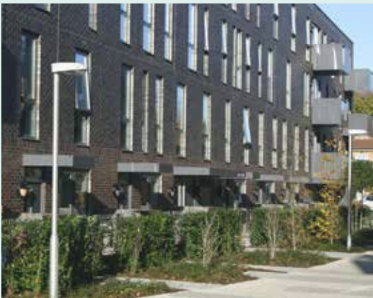
Front garden amenity as buffer between public paths and maisonette front door
