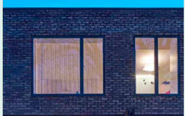
Window opening with no brick reveal
