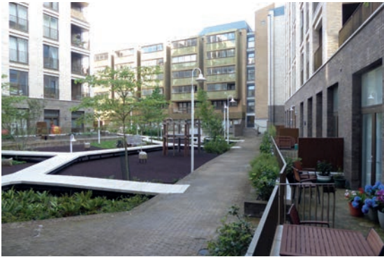
Easy connection between ground floor doors and courtyard play spaces. (Source: Publica)
