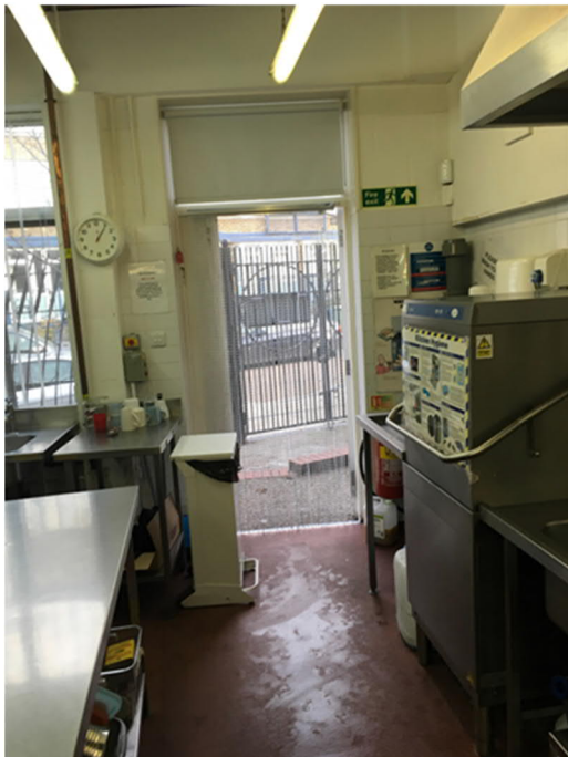
Kitchen with doors open to provide ventilation as mechanical ventilation is not working
