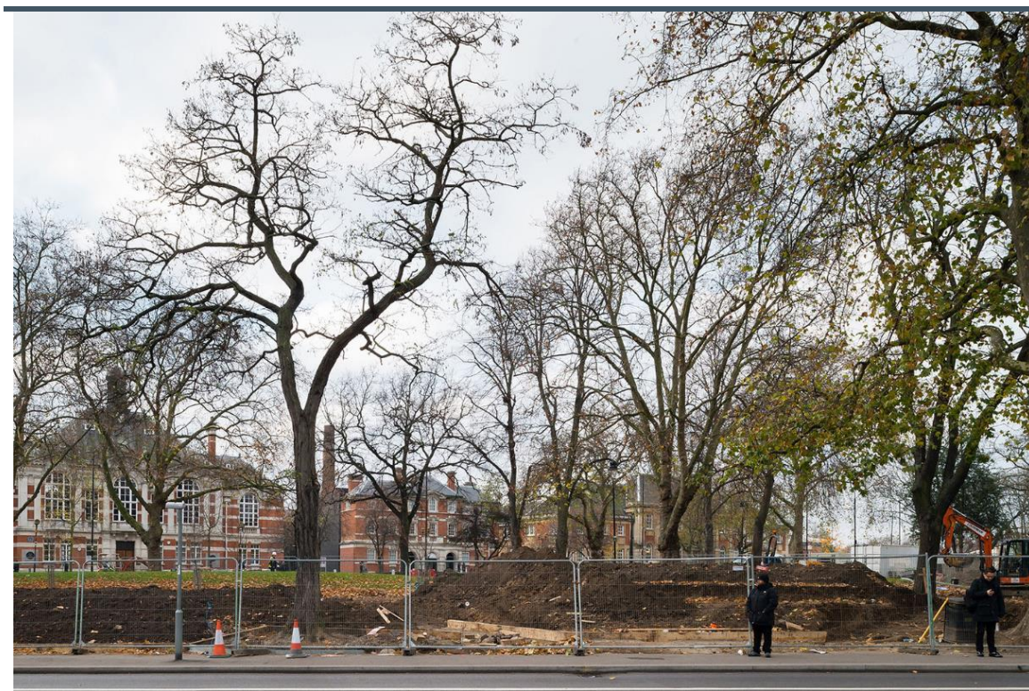
Works on Tottenham Green
