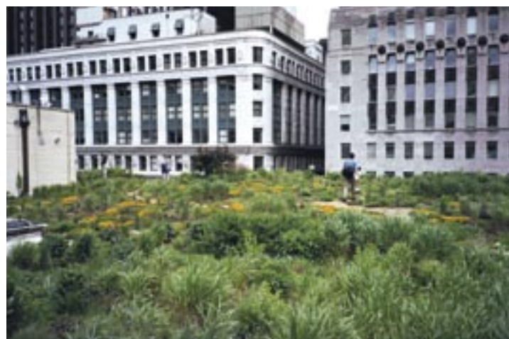
Green Roof, Chicago City Hall One of first to be installed in programme to reduce UHIE. Photo: Mathew Frith
