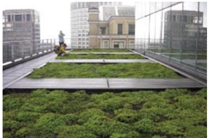
Extensive Roofs don't have to be restricted access Canary Wharf – sedum plug roof. Photo: Livingroofs.org
