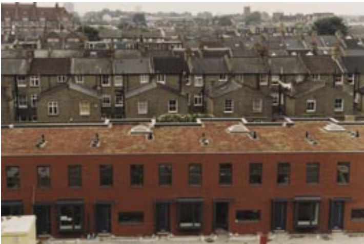
Sedum Roof, Lille Road. Photo: Mathew Frith
