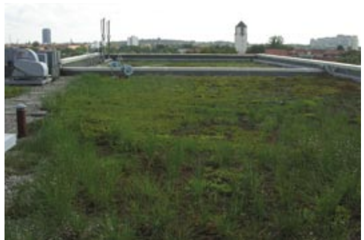
Sedum/Herb Roof Berlin. Photo: Livingroofs.org
