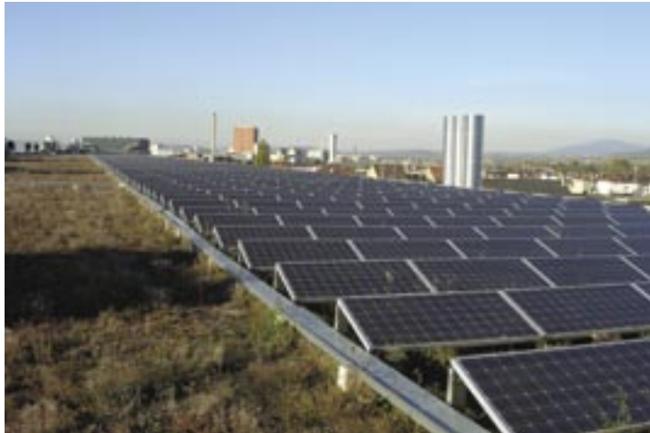
Largest A Frame PV Roof in Europe on a green roof, Switzerland. Photo: Livingroofs.org
