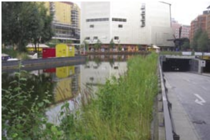
Part Roof Lake used to recycled water Potsdamer Platz, Berlin. Photo: Livingroofs.org
