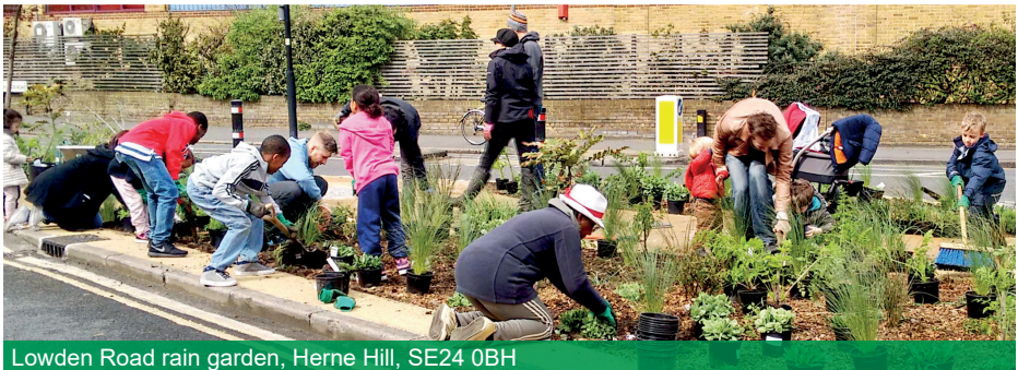
Lowden Road rain garden, Herne Hill, SE24 0BH
